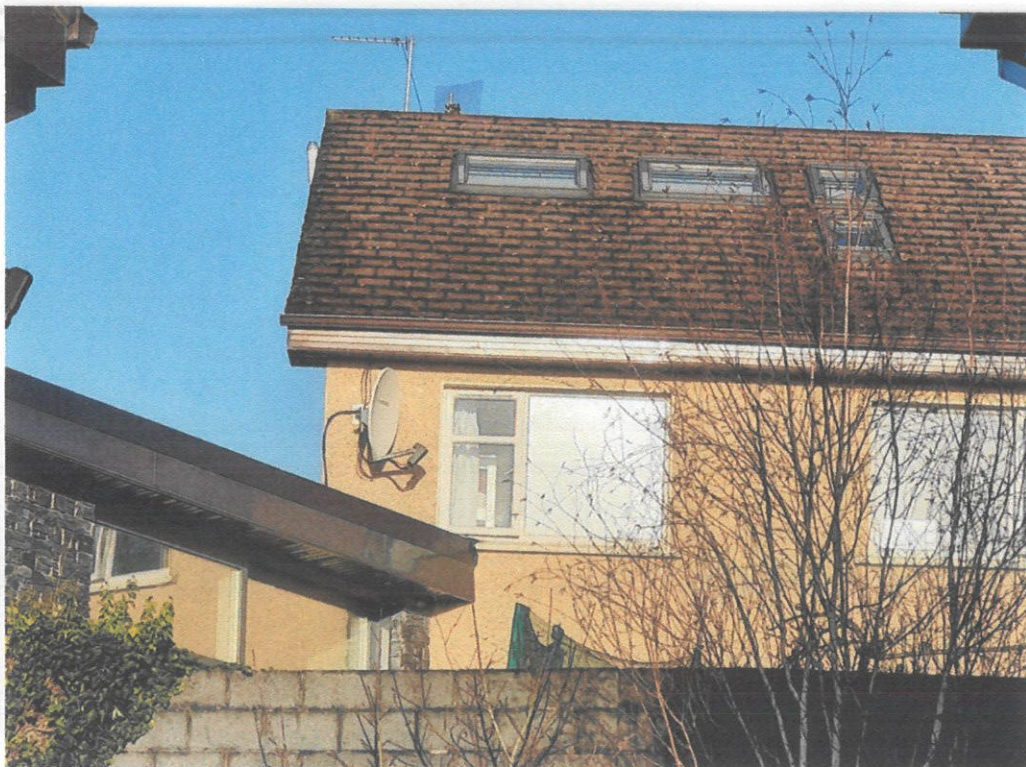
Picture 6: Showing velux rooflights to the rear.
